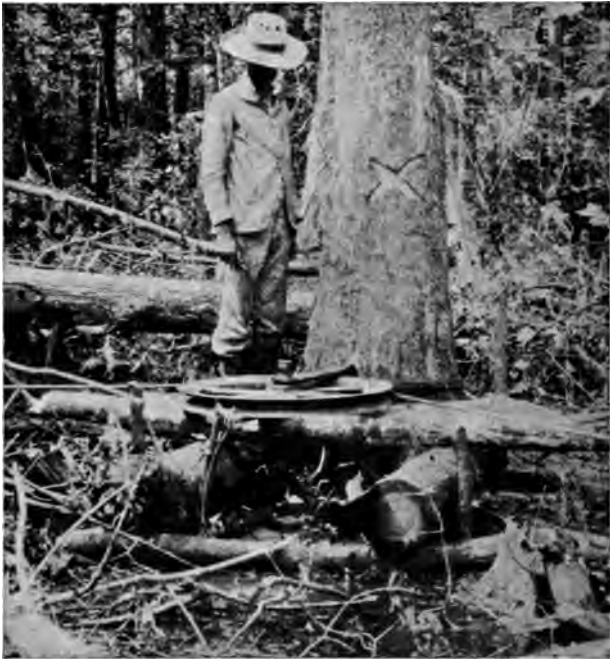
FIG. 59. — The Sheave Block attached to the Tail Tree. Note the method of supporting the block.
